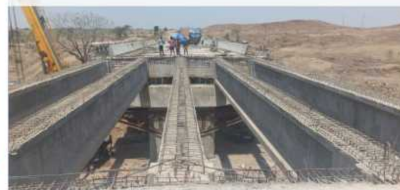
This Project includes One Major Bridge having 4 spans Each Span is of 25 meters. Total Length of Bridge is 100 meters. It is Precast RCC Girder Bridge.
