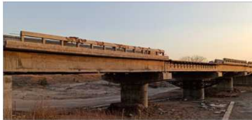
This Project includes One Major Bridge having 4 spans Each Span is of 25 meters. Total Length of Bridge is 100 meters. It is Precast RCC Girder Bridge.
