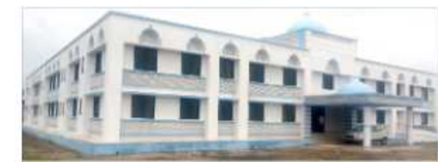
100 Student Hostel Building of Social Justice Department at Shindkheda, Dhule
