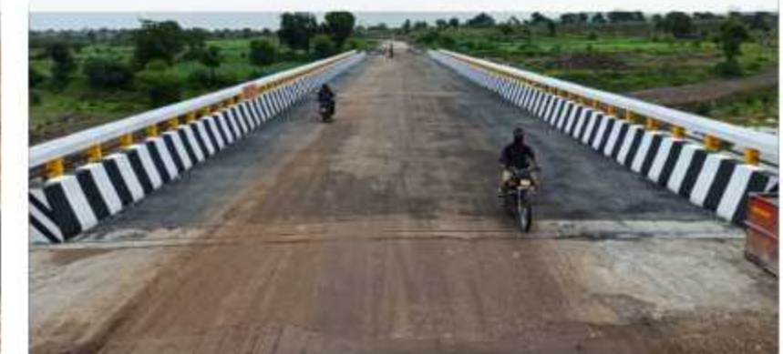
This Project includes One Major Bridge having 4 spans Each Span is of 25 meters. Total Length of Bridge is 100 meters. It is Precast RCC Girder Bridge.
