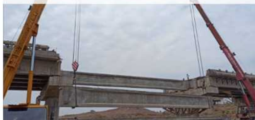
This Project includes One Major Bridge having 4 spans Each Span is of 25 meters. Total Length of Bridge is 100 meters. It is Precast RCC Girder Bridge.
