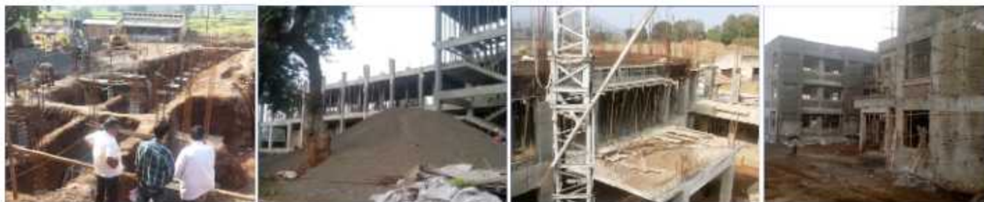
Construction of Ashram School Building at Bapkheda, Kalwan, Nashik
