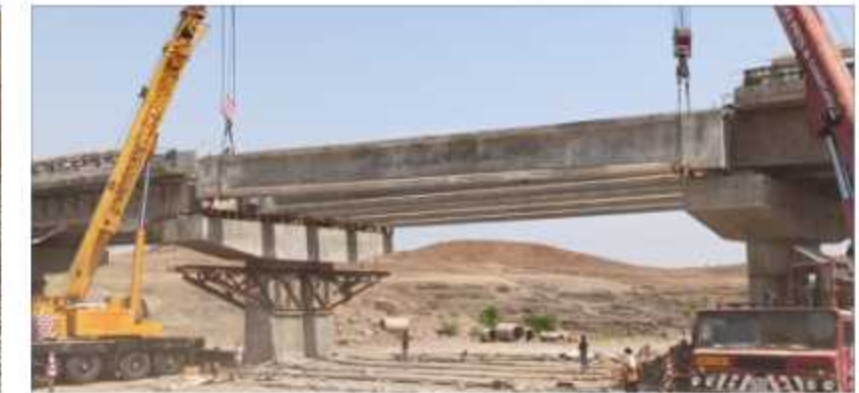
This Project includes One Major Bridge having 4 spans Each Span is of 25 meters. Total Length of Bridge is 100 meters. It is Precast RCC Girder Bridge.
