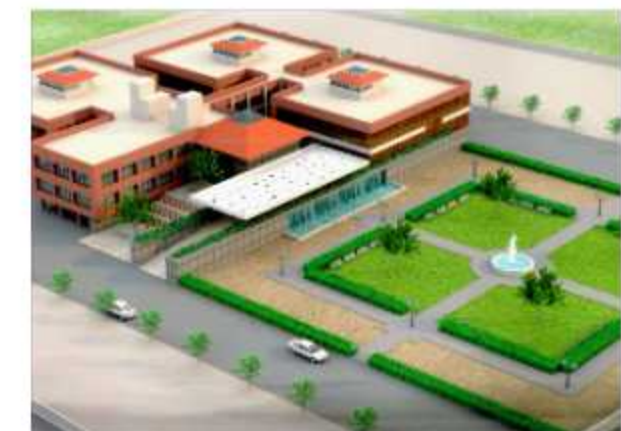
Dhule, Municipal Corporation Administrative Building
