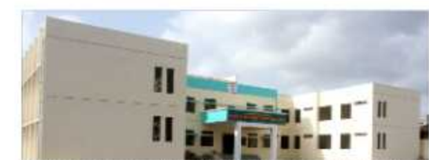
Construction of Ashram School Building at Bandarpoda, Kalwan, Nashik
